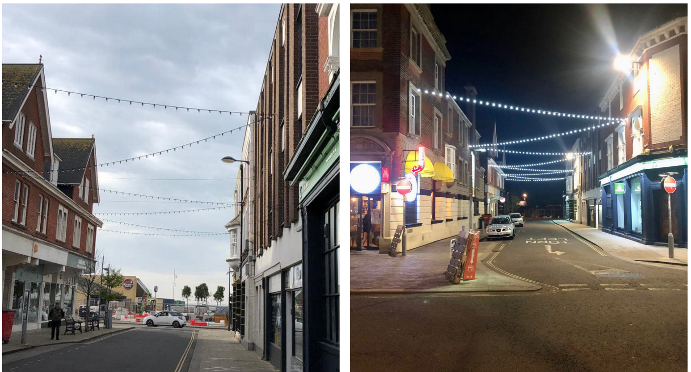
Welcoming Town: Fantastic news - festoon lighting has been installed at York Road - this is a partnership project, with Bognor Regis businesses delivering the lights and maintenance through BID levy payments, and electrical supply provided by Arun District Council.
